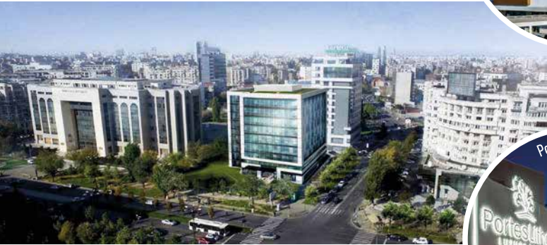
Day Tower - Office Building - Bucharest
